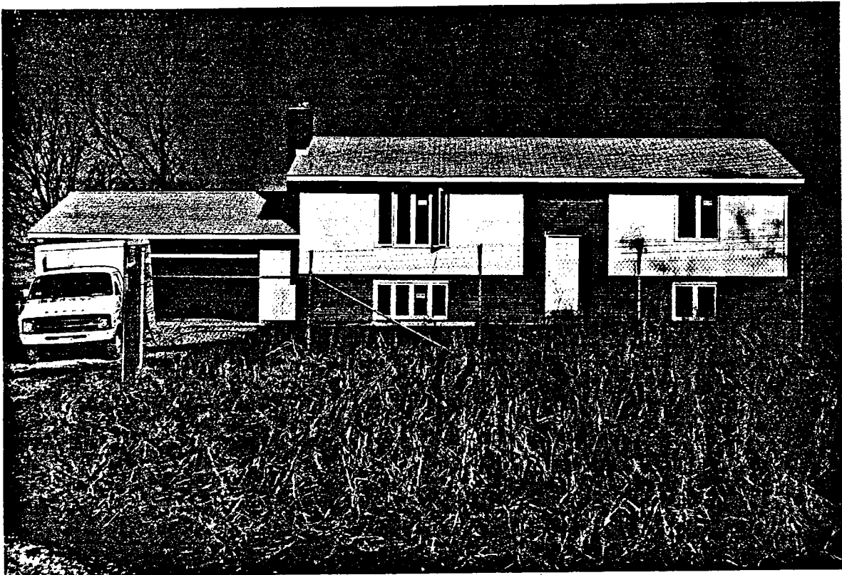
Figure 42.—Test residential fatigue structure near surface coal mine. ANRSHIAE
