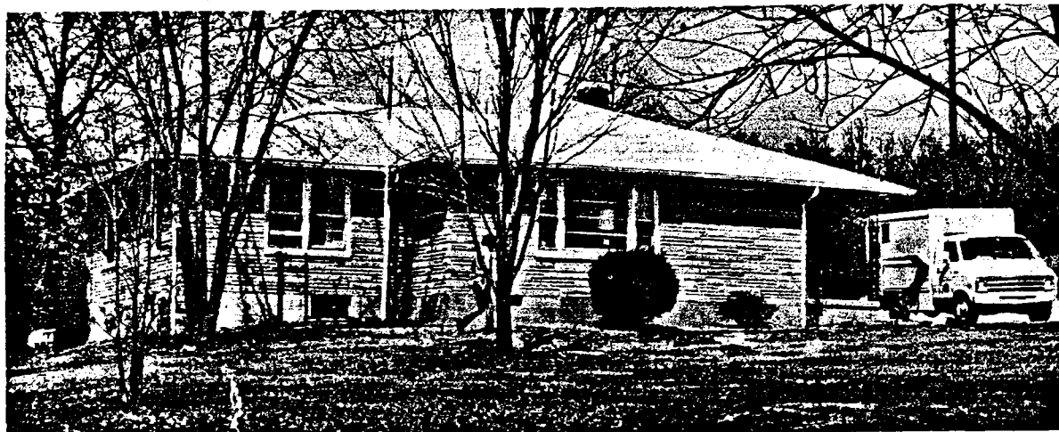
Figure 24.—Test structure 30, near a coal mine.
