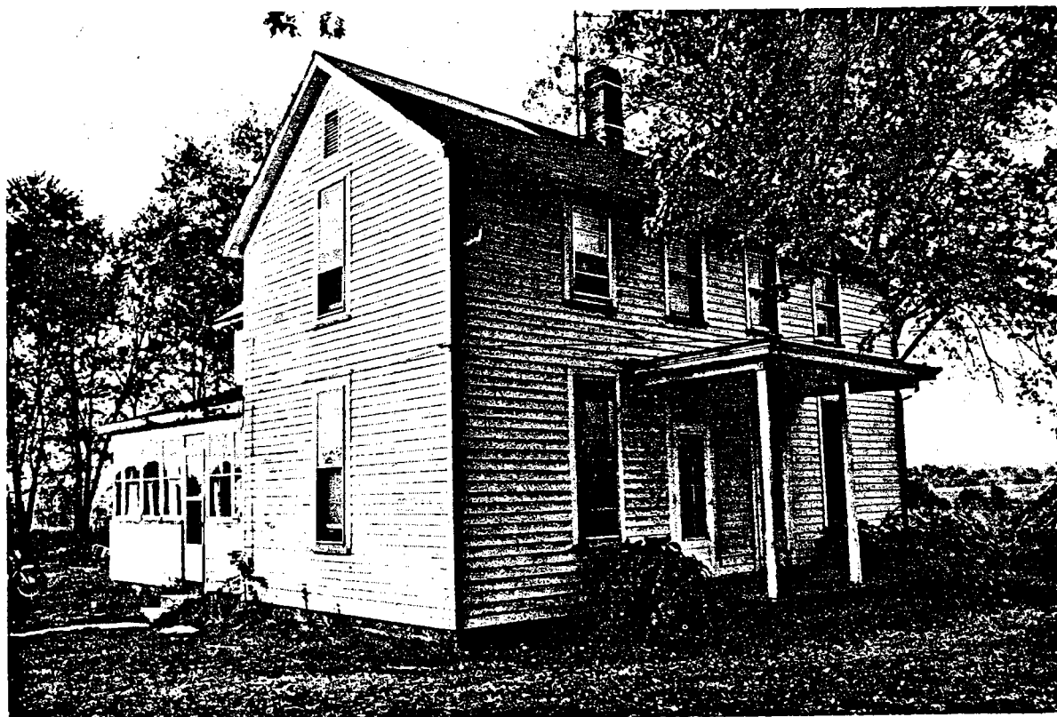
Figure 15.—Test structure 19, near a coal mine.
