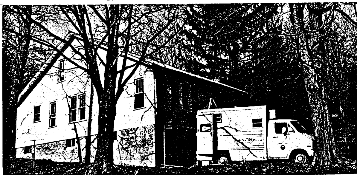
Figure 26.—Test structure 49, near a coal mine.
