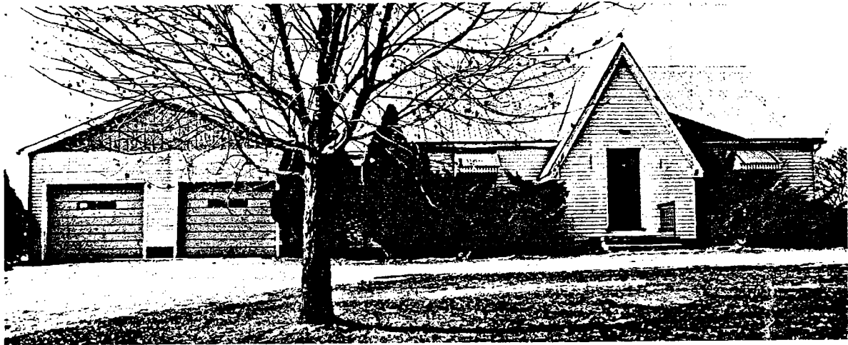
Figure 16.—Test structure 20, near a coal mine.
