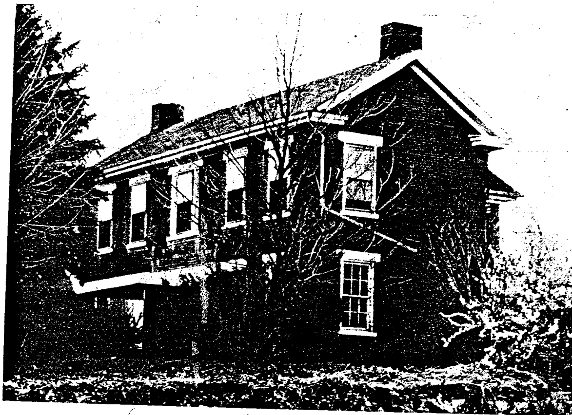
Figure 27.—Test structure 51, near a coal mine.
